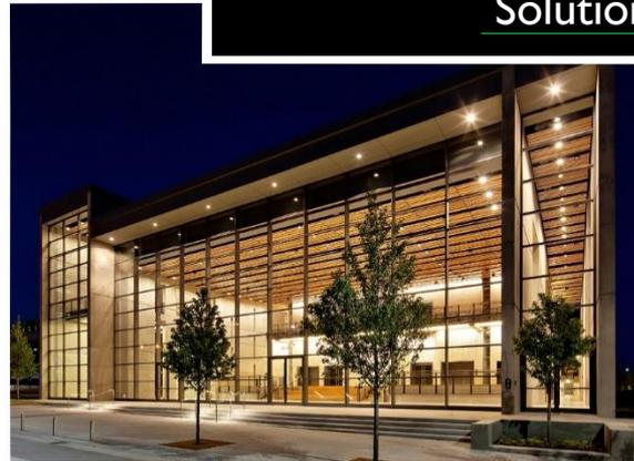
Montanstahl was able to manufacture the extra-long mullions by first laser-cutting strips from steel plates and then laser-welding them to the desired hollow sections, thereby meeting the structural requirements while allowing great design flexibility.
